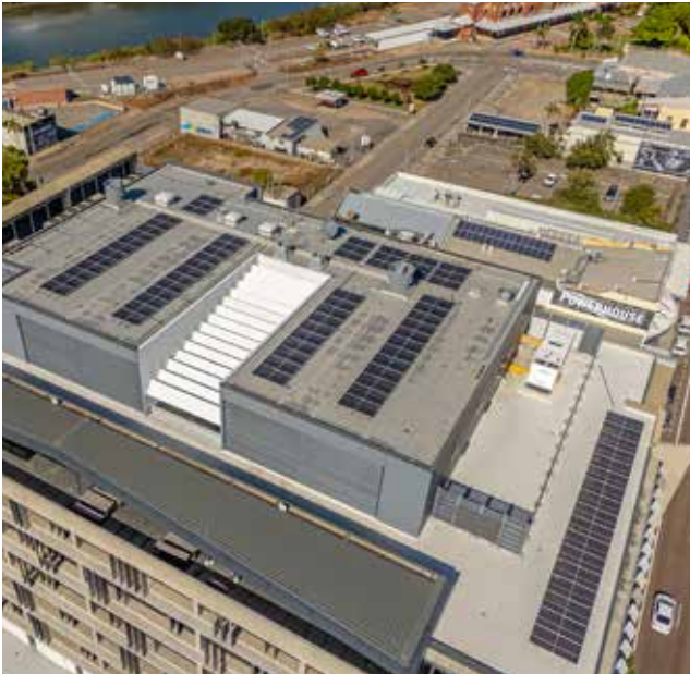
Solar works at 420 Flinders Street, Townsville
